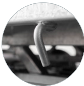
Long tie-hooks under the floor
